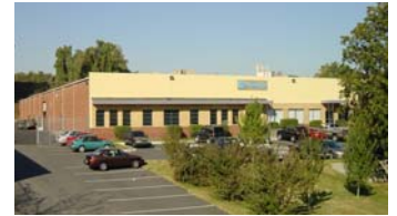
View of Coldwater Seals, Inc. from Chattahoochee Ave
